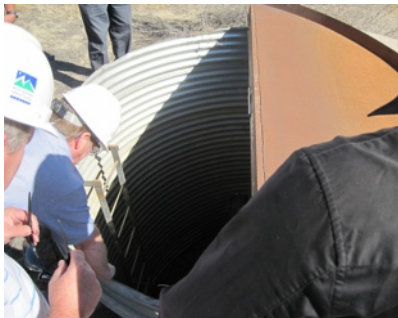
STWA CEO, Cecil Bond Kyte looks on as U.S. Department Of Energy contractor field operations personnel showcase one of the bell holes.
